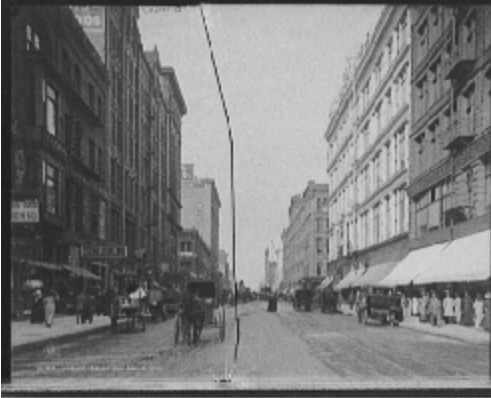
Nicollet Avenue, Minneapolis, Minnesota
