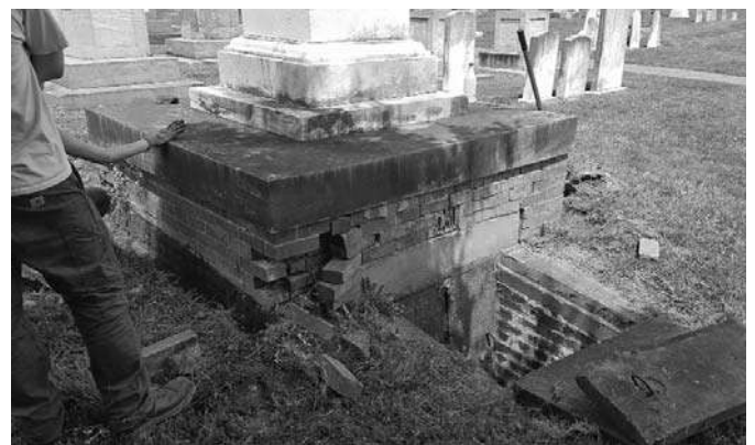
Hyatt Vault before.
