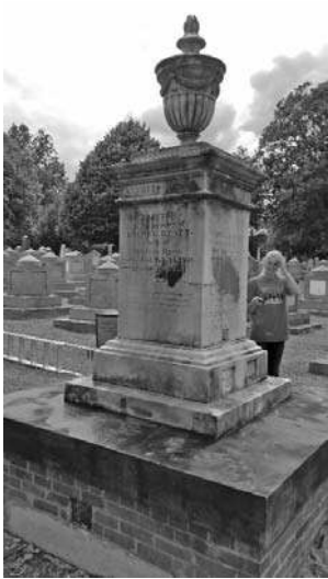
Hyatt Vault during.
