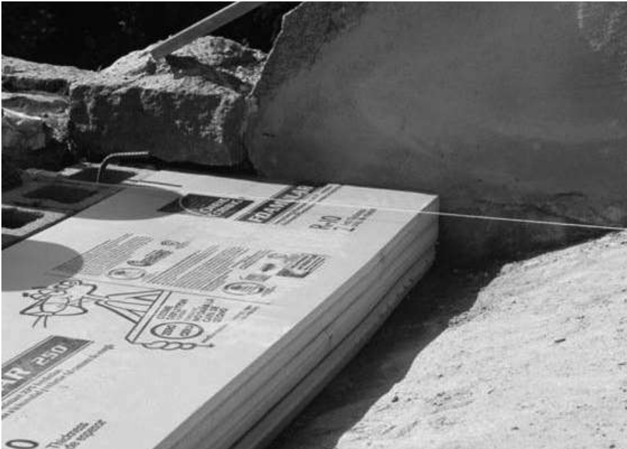
Polystyrene blocks to reduce the burden on the barrel vaults.
