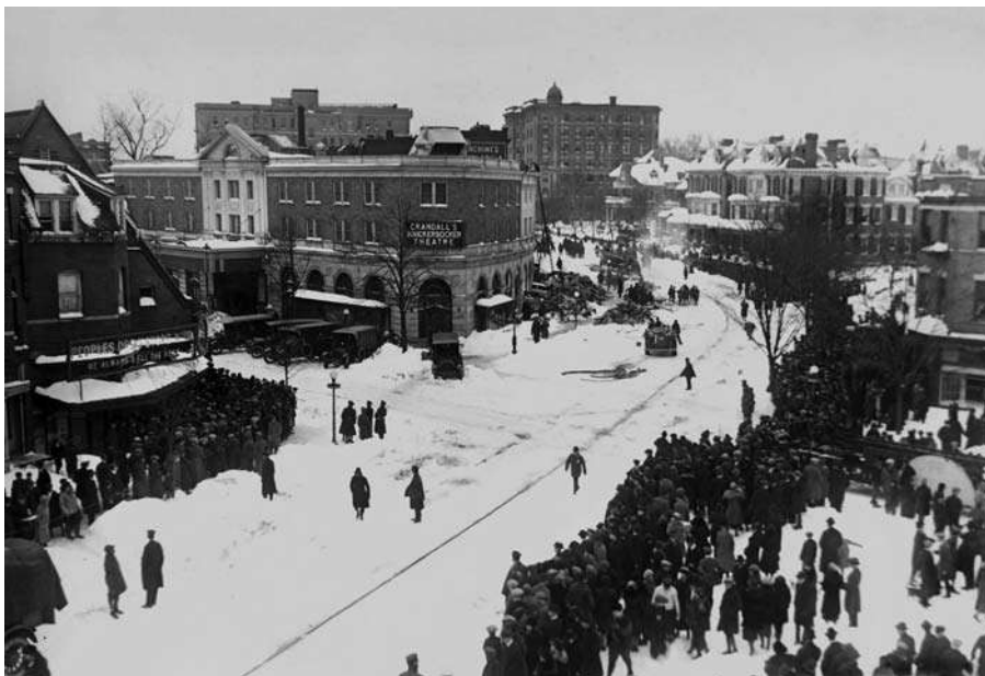
Knickerbocker Theatre during recovery efforts.
