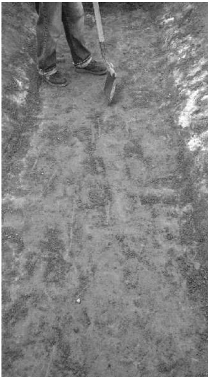
Fill above the barrel vault.
