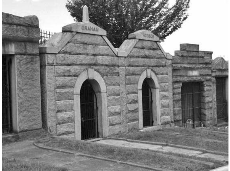
Graham and Hodges Mausoleums after cleaning.
