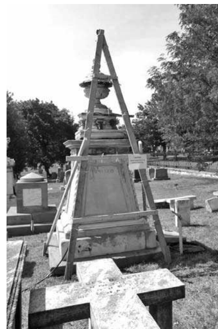
Restoration of the Gerry monument
