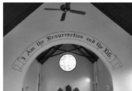
The restored Chapel wall
