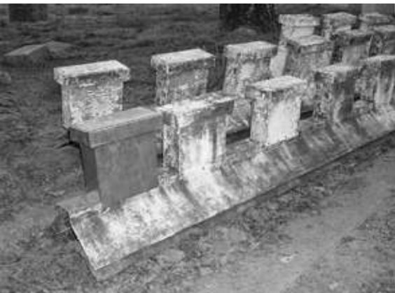
Roof ridge cresting is brought down for repairs.
