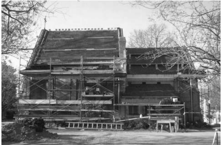
The chapel undergoes a roof renovation with replacement Buckingham slate.
