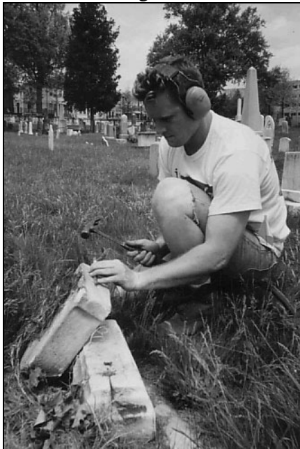
Removing rusted pins
