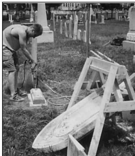
Drilling support shafts
