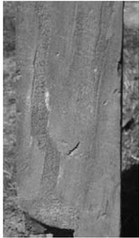
Although the mortar was color-matched to aid in concealing the repair from a distance, it is easy to distinguish from the sandstone.
