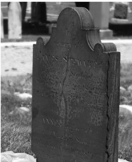
*With such severe delamination, detachment and loss of material were inevitable.*
