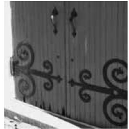
eliminate this is the future, but the doors must be replaced to prevent further damage to the interior floor of the chapel.
